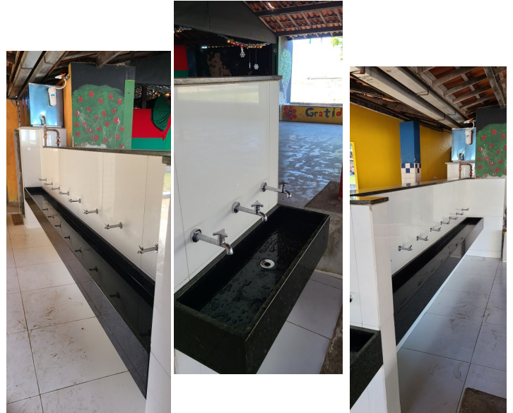
The new water fountain has 8 spigots on each side and 3 taps for filling water bottles.
